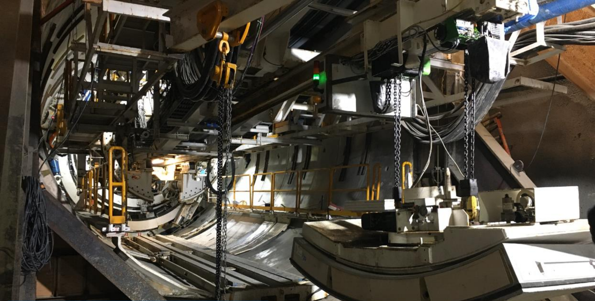
Initial TBM Advance & PCTL Installation
